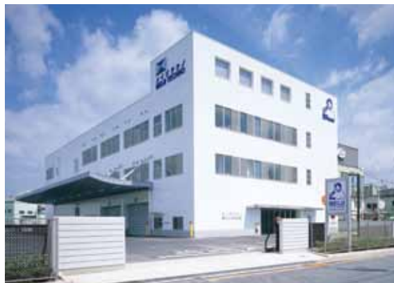
Head office · Factory (Miyoshi-machi, Saitama, Japan)
